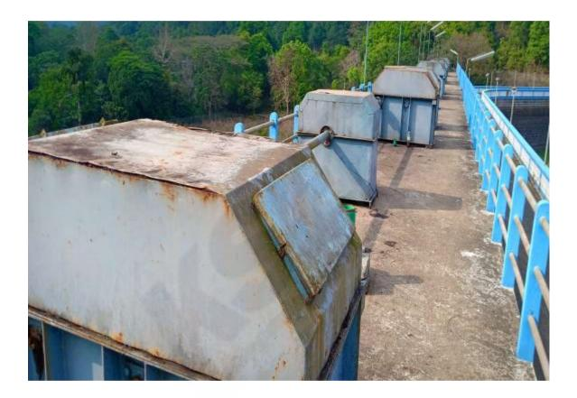
Fig 2.5 Radial gate Hoists
