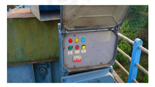
Fig 2.7 Control panel of Hoisting mechanism
