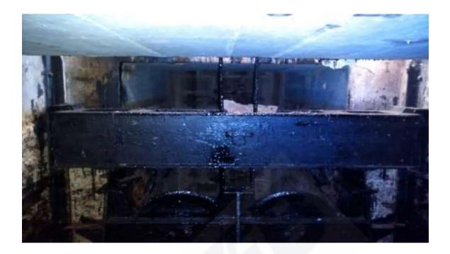
Fig 6.3 Emergency gate guides before replacement
