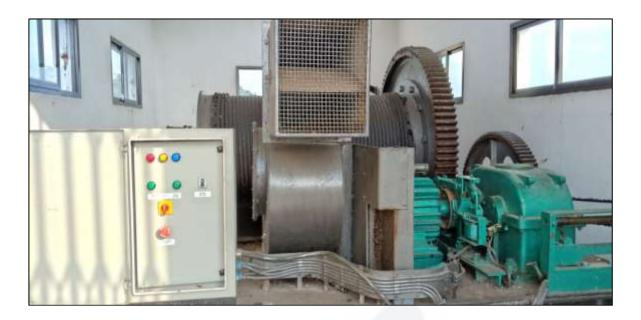
Fig 2.15 Rope drum of Emergency gate
