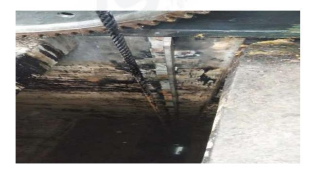
Fig 6.4 Emergency gate guide after replacement
