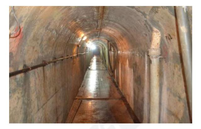
Fig 2.9 Drainage and inspection gallery
